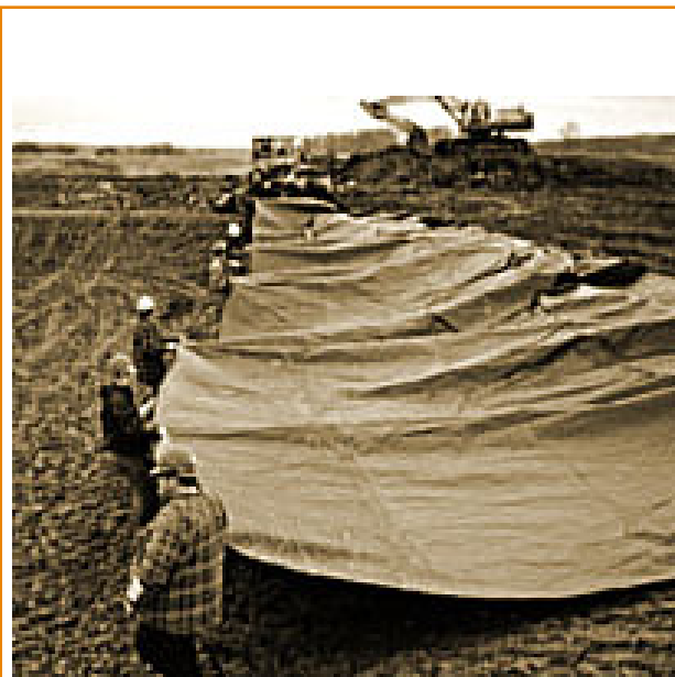
Pulling out a Fabricated Geomembrane Panel
